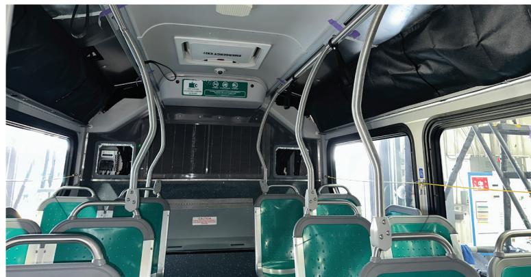
During final assembly, every detail counted - even ensuring the signature green seats were perfectly installed.
