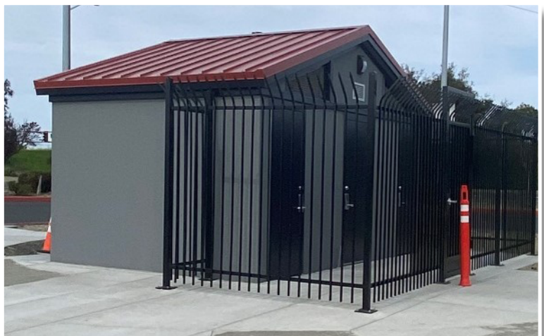
The entrance to the two-unit restroom is secured by a fence and a locking gate, which will be equipped with card reader badge access.
