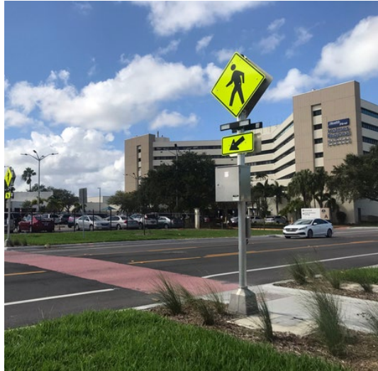
Rectangular Flashing Beacons
