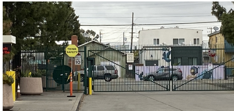
Integrated with new badge security systems, upgraded gates create a more secure workplace, enhancing morale and job satisfaction.
