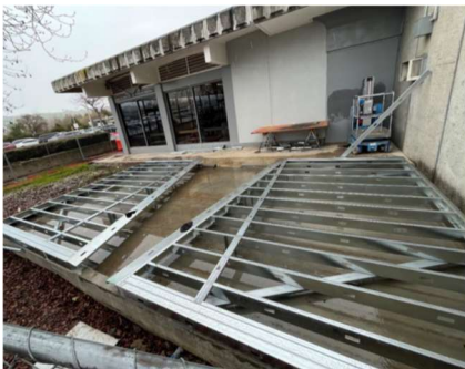
Two Walls on Pad 03-13-2023
