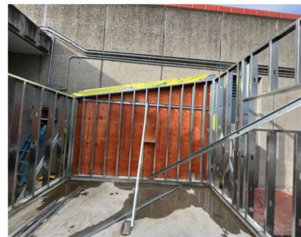
Three Walls Up 03-27-2023
