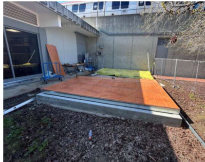
Two Walls Sheathed 03-20-2023
