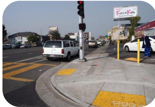
ADA ramp upgrades
