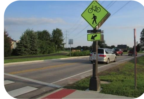
Flashing Beacons (RRFBs)
