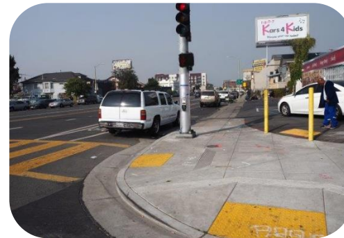
ADA ramp and signal upgrades
