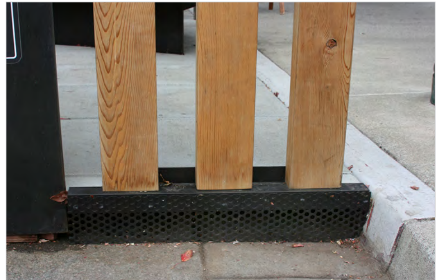
Gutter grate and Drainage treatment at the Pilot Bus Parklet in Albany
