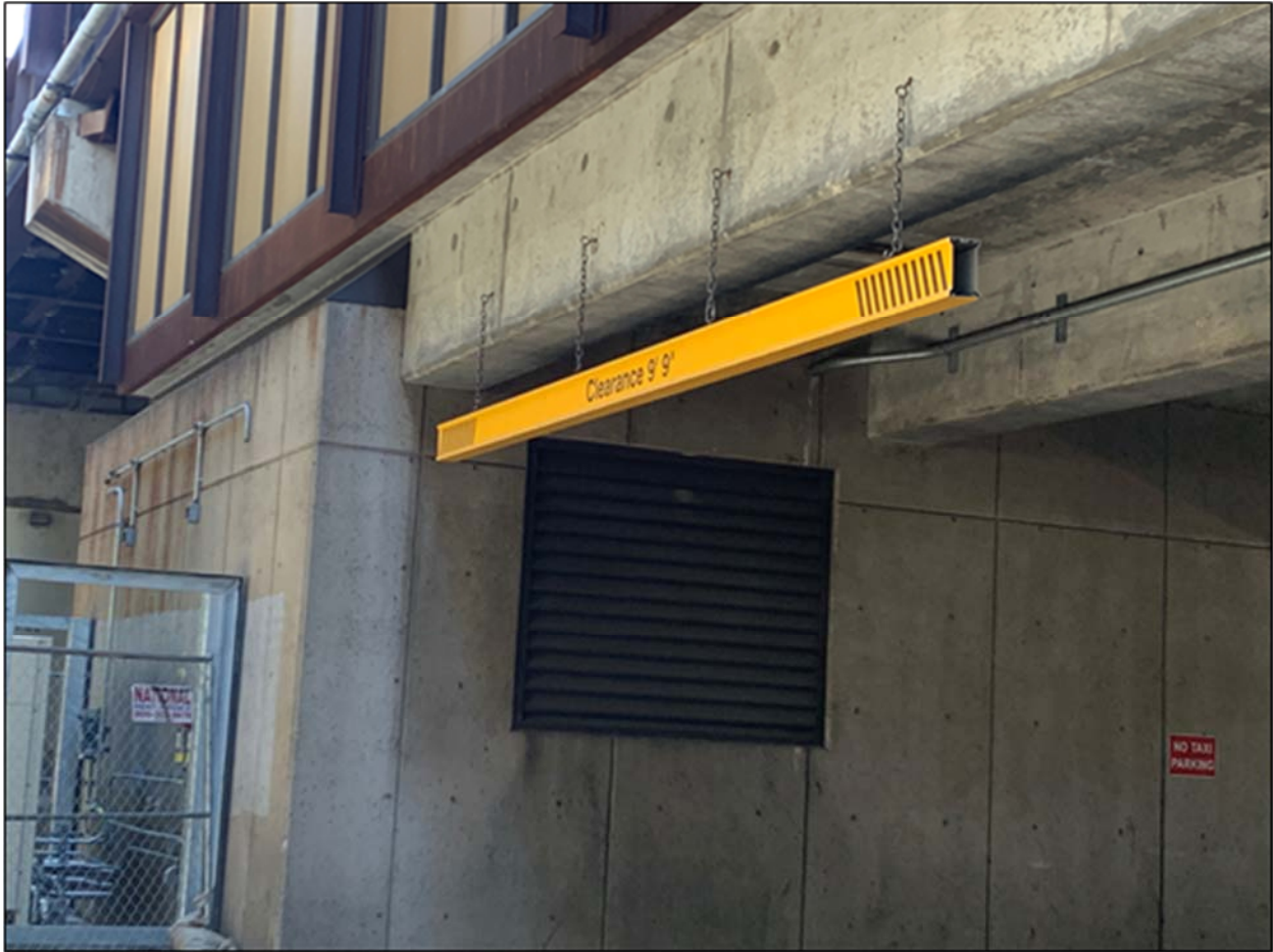
Exhibit 15 - Rockridge BART Station Internal Roadway Clearance Sign
