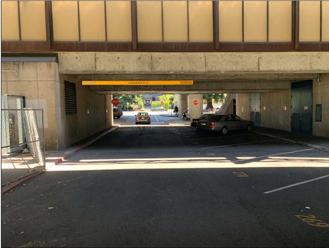
Exhibit 5 - Internal Roadway at Rockridge BART Station (looking south)
