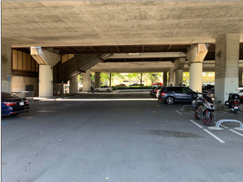
Exhibit 11 – Rockridge BART Station Parking Lot- Eastside (looking north)
