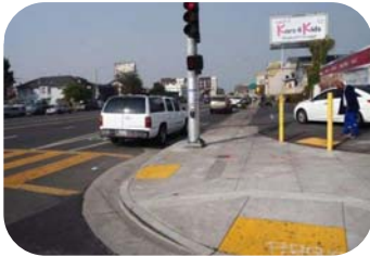
ADA ramp and signal upgrades
