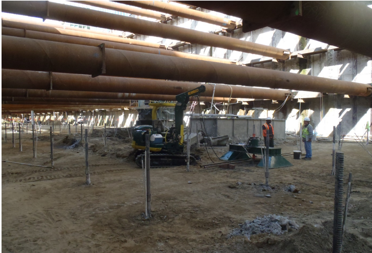
Micropile Pull Test Underway
