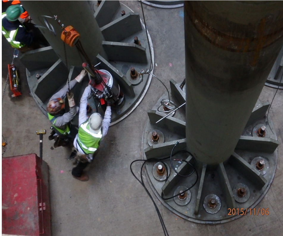
Bolt tensioning underway at Light Column
