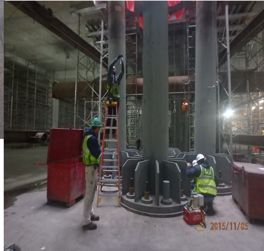
Bolt Tensioning Inspection
