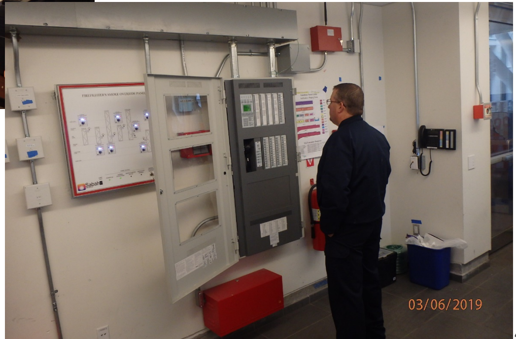
Building Fire Alarm Panel
